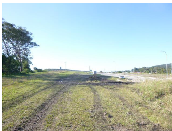
Looking north east from Lot 73 showing grass cover and gentle slopes within stage 1B
