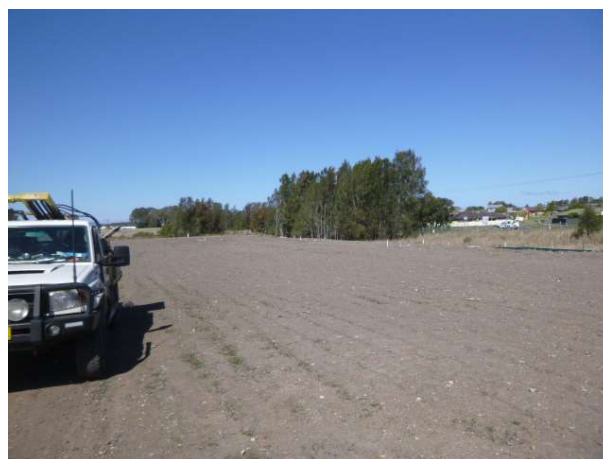
View south east from Lot 96 showing flat to gentle slopes on this area which has been regraded by placement of fill.
